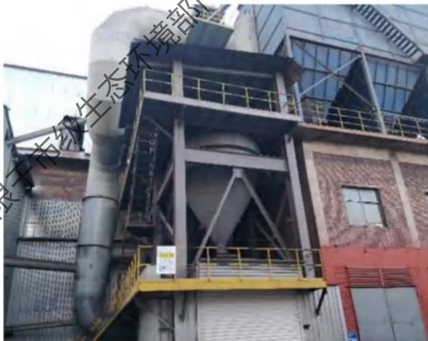
2#矿槽除尘灰筒仓
